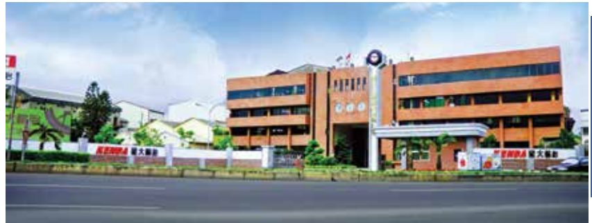
The Kenda headquarters in Taiwan.
