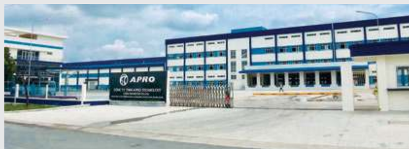
When A-Pro's new factory in Vietnam's Binh Duong province is fully operational this year, it will have a workforce of about 500.
