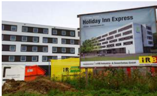
Holiday Inn Express under construction.
