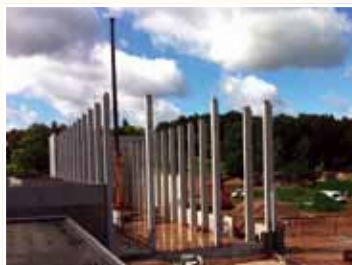
CONSTRUCTION OF THE NEW LOGISTICS CENTER.
